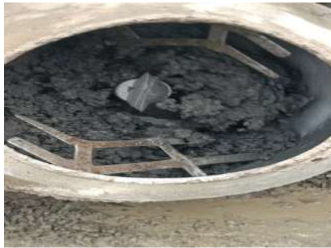
Fig. 6 Mixing of material in concrete Mixer
